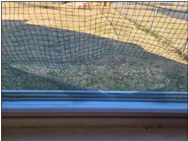
3.6 Item 1(Picture) Window exterior screens-damaged
