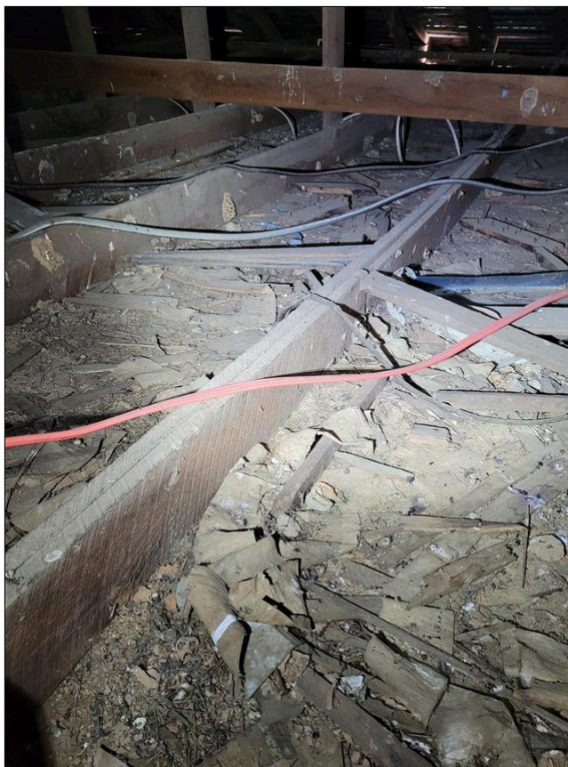
4.3 Item 2(Picture) 1"x6" ceiling joists
