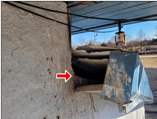
2.4 Item 1(Picture) Open soffit area
