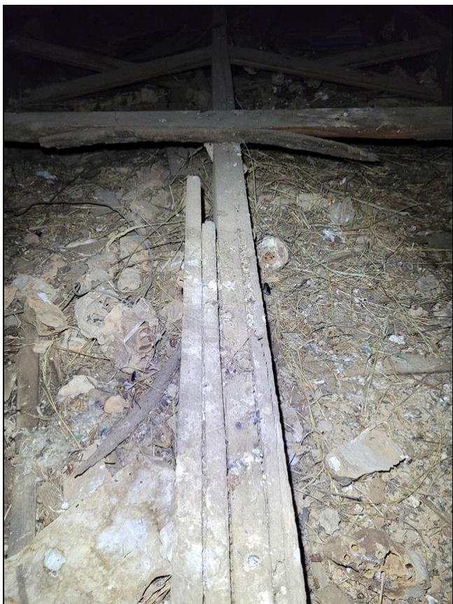
4.3 Item 1(Picture) 1"x6" ceiling joists
