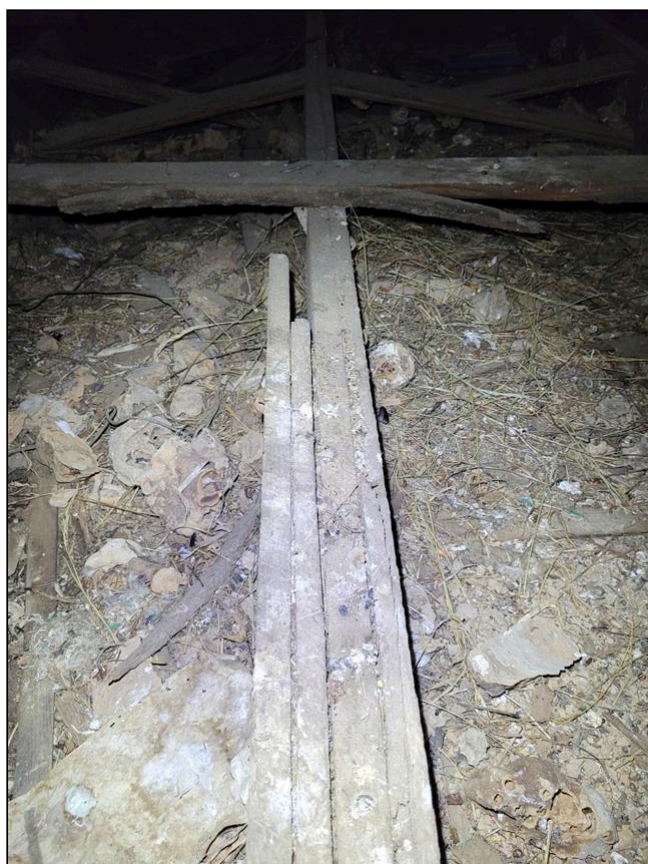
4.3 Item 1(Picture) 1"x6" ceiling joists
