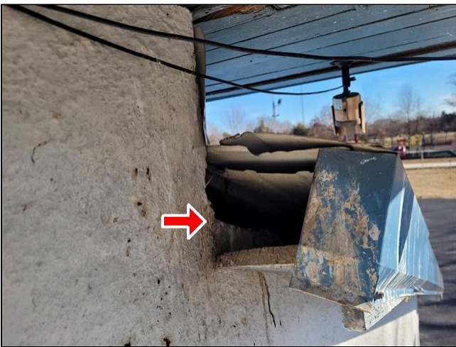
2.4 Item 1(Picture) Open soffit area
