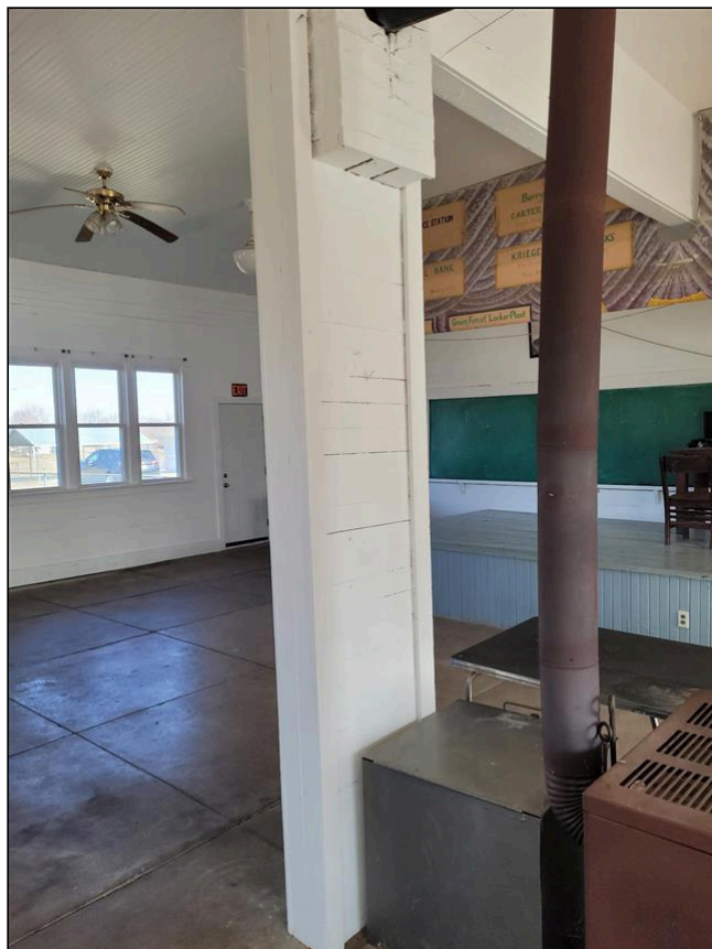
7.3 Item 1(Picture) Removed brick chimney
