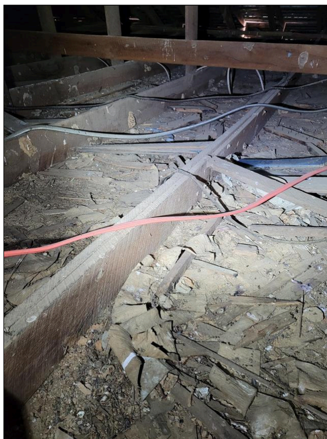
4.3 Item 2(Picture) 1"x6" ceiling joists
