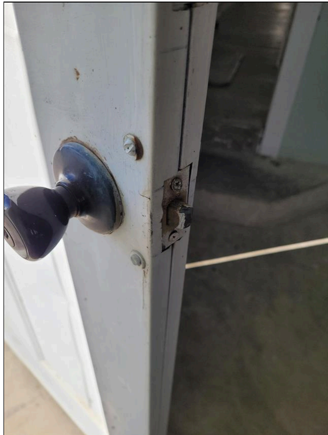
2.1 Item 4(Picture) Repaired door-Southwest side
