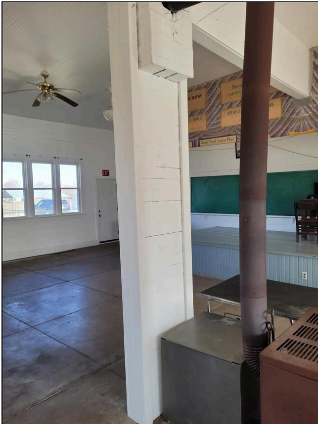
7.3 Item 1(Picture) Removed brick chimney
